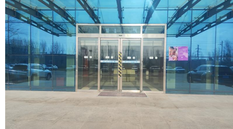
An example of vinyl safety dots used on the doors to reception in our Chifeng, China site.
